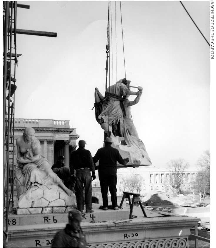
Fig. 2. Lifting north section of Rescue from upper north cheek block.
