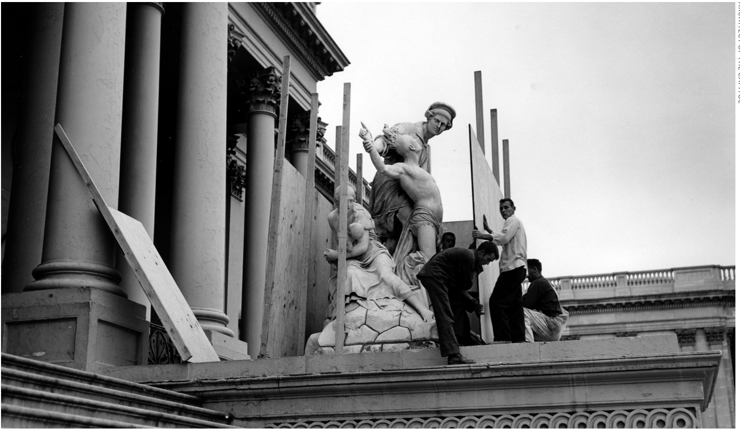
Fig. 3. Crating Rescue on upper north cheek block.
