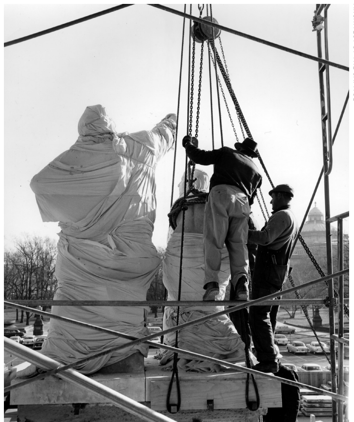
Fig. 5. View showing Discovery group being safely removed from the upper south cheek block of the central steps on Nov. 25, 1958.
